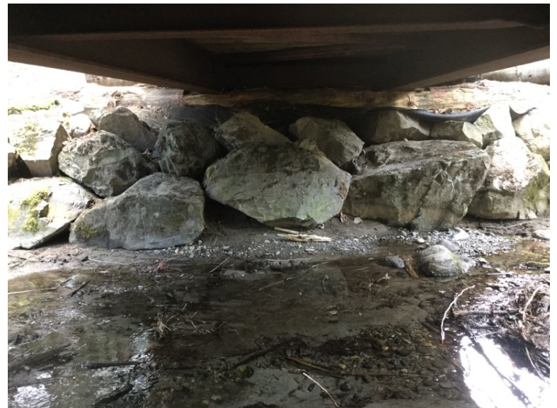
Left Bank Abutment when facing downstream
