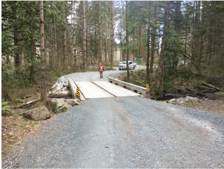
Approach from Left Bank when facing downstream
