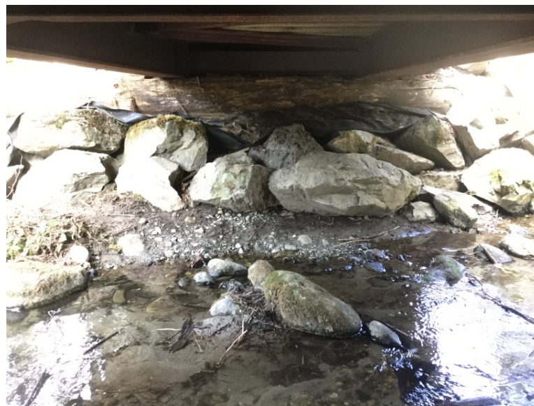
Right Bank Abutment when facing downstream
